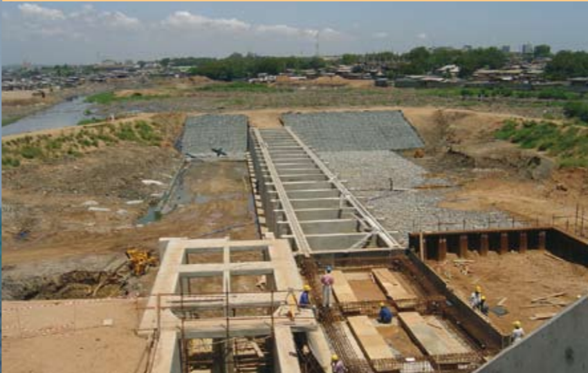
Construction of the interceptor for the "Korle Lagoon Ecological Restoration Project", Ghana
