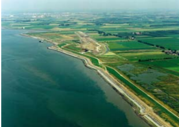
Dike construction, Ellewoutsdijk, The Netherlands.
