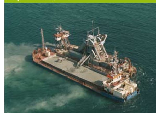
Bucket Dredger "Ajax R" loading soil into Hopper Barge "Magni R". This project which was finished early in 2005 involved moving, re-use and utilisation of 200.000 m 3 soft and hard soil from the dredged channel to the enlarged Port of Grenaa, Denmark.
