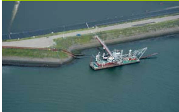
Barge unloading system at the Werkhaven sludge recycling centre.
