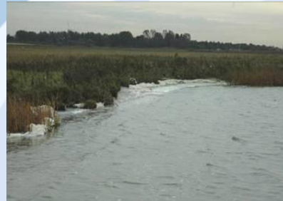
IJsselmeer foreshore nourishment
