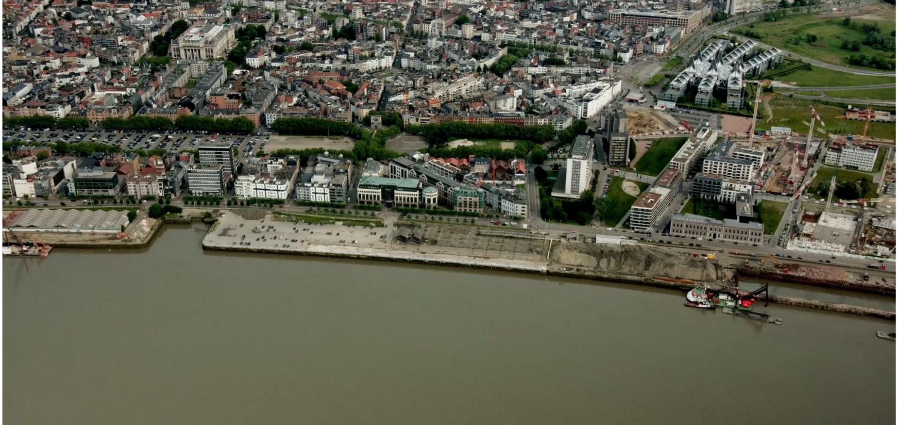
Innovative approach Stabilisation techniques of the quays in Antwerp
